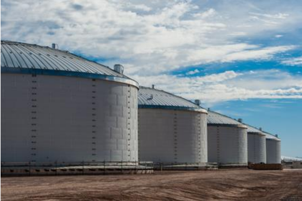
Solana Generating Station (2013, U.S., ~4200 MWh(t))
