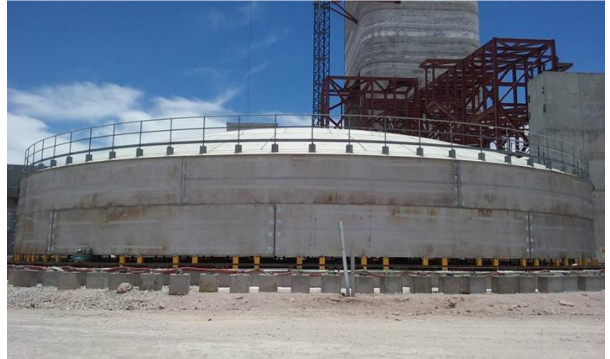
Cerro Dominador Project ( under construction , Chile, ~4800 MWh(t))
